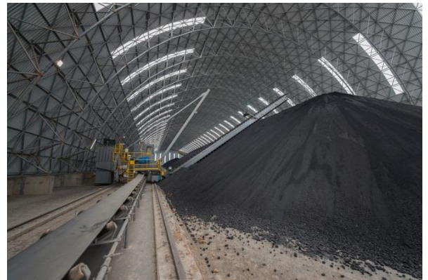
Coal storage warehouse
